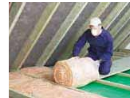
Figure 3 Insulating a loft. The air trapped between fibres make fibreglass a good thermal insulator.
