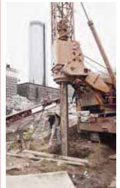
Figure 4 A pile driver in action
